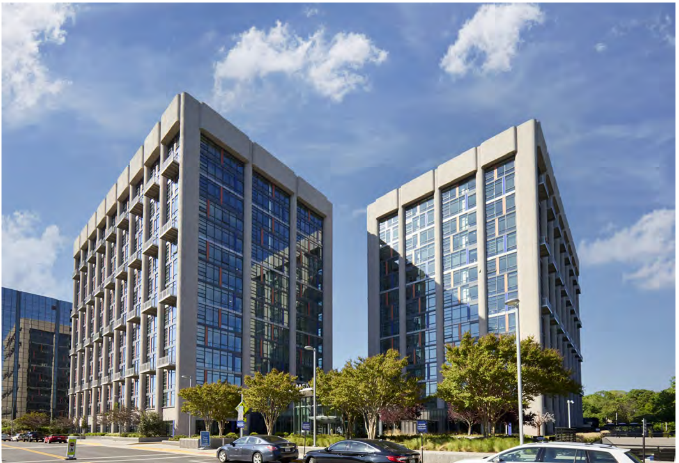
An example of a successful recent office to residential conversion - Park Ford. Though it is possible, there are significant challenges involved when converting office to residential.
