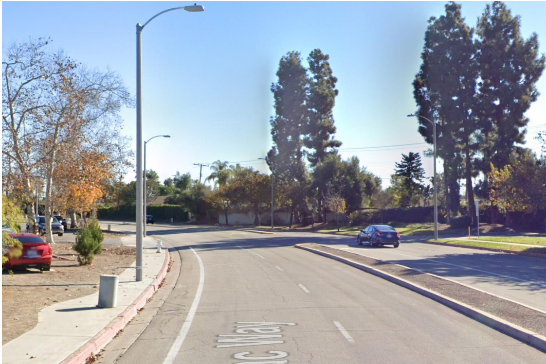
Merrimac Way, Before
