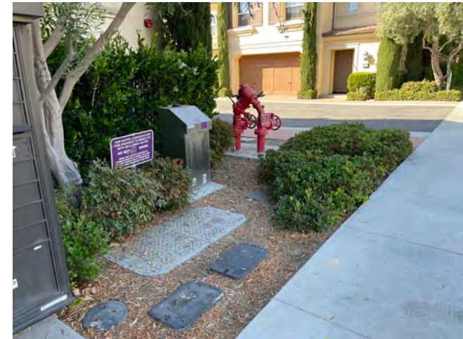
Planting shall maintain the minimum clearance when it is close to the utility facilities and fire hydrants.
