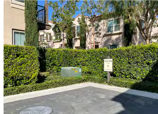
Mechanical equipment shall be either placed on the ground and screened with landscape.
