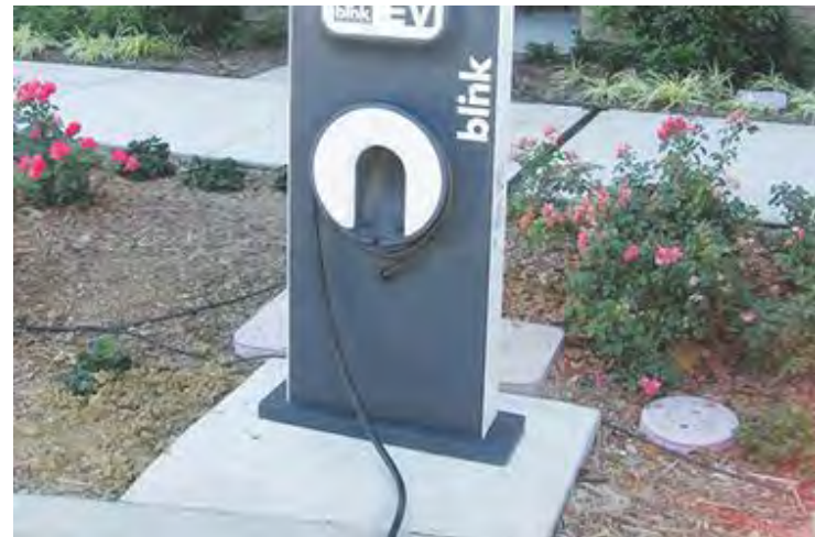
Standard 2.12.d: Charging station shall be a minimum of 24 inches clear from the face of curb.
