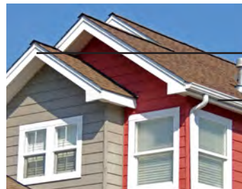
Rake Overhanging Eave Overhanging
